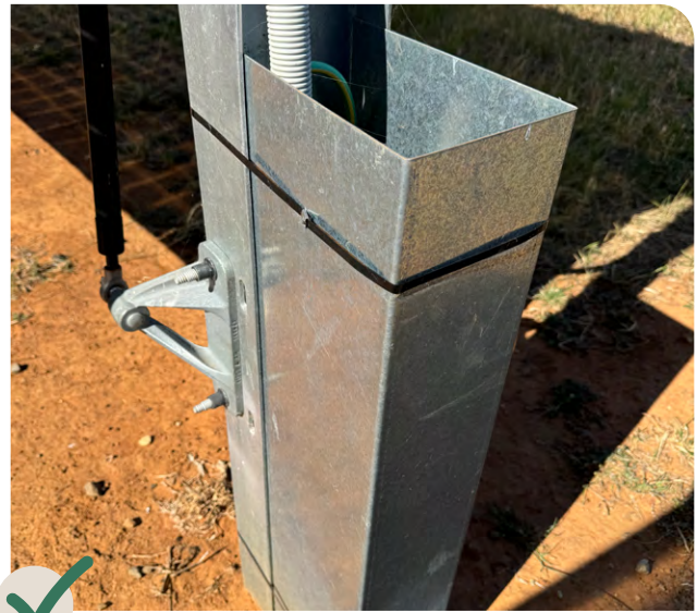
Protective guard to prevent sheep damage
