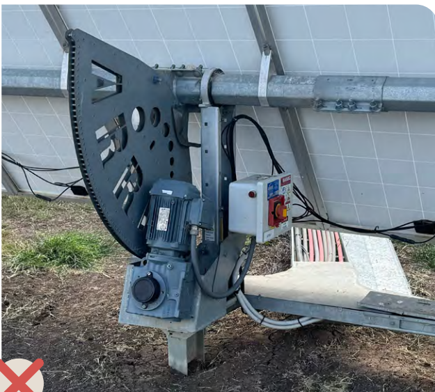
Exposed equipment accessible to sheep
