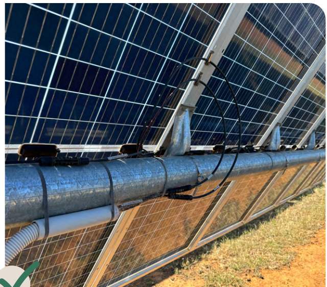
Wires inaccessible to sheep
