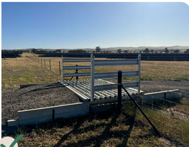
Retrofitted internal fencing and access grid
