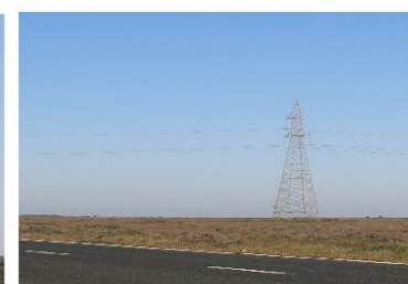
Cables extending across the view
