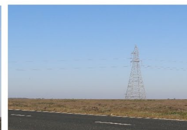
Cables extending across the view
