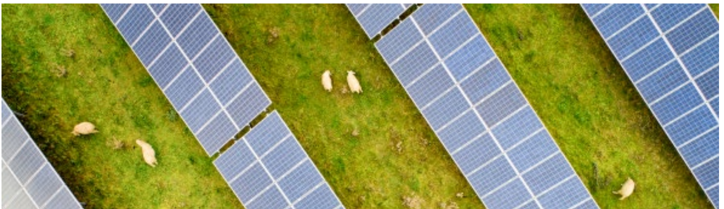
High angle view of solar panels.
