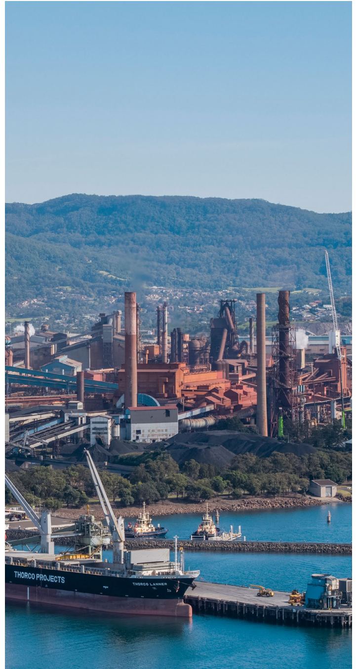
Image courtesy of NSW Department of Planning and Environment. Portside factories, Port Kembla.
