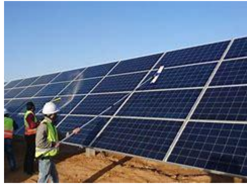
Cleaning PV solar panels
