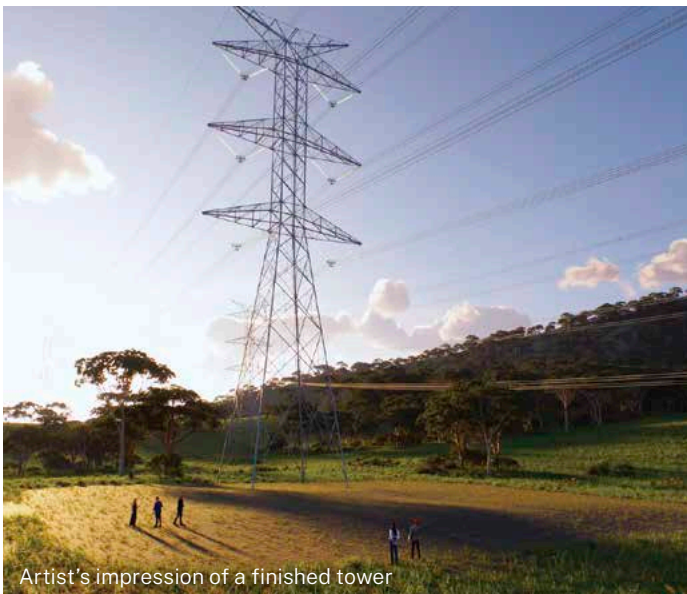
Different types of transmission infrastructure
